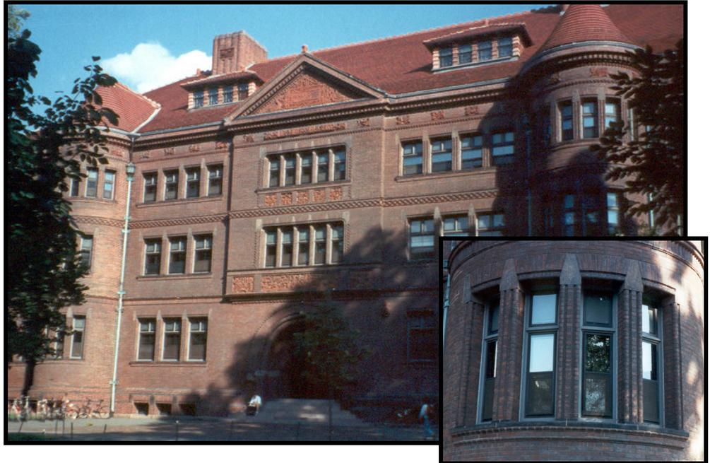
*Sever Hall, in the heart of Harvard yard, was made more energy efficient by installation of new storm windows. However to avoid a "new" look for the building, the windows have a black anodized aluminum finish to retain the old traditional appearance of the building.*
